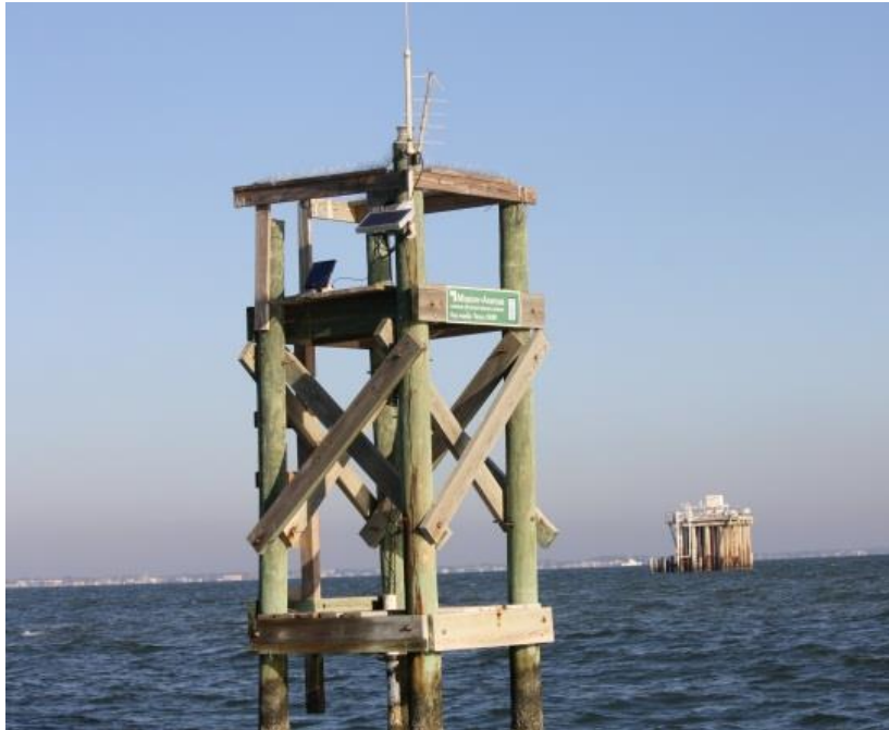
Mission-Aransas NERR SWMP station
